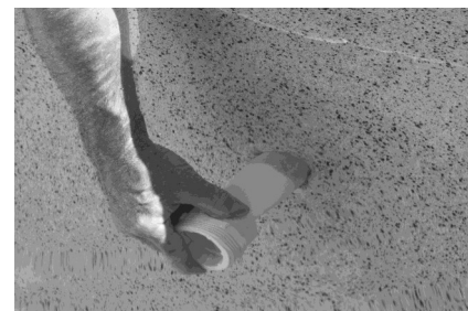
Push in Sanded Insert (1) into hole
