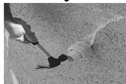
Tap in the Bung (5) into Sanded Insert (1). This will open the sanded end of the Sanded Insert and secure it to the inside of the pool return.
