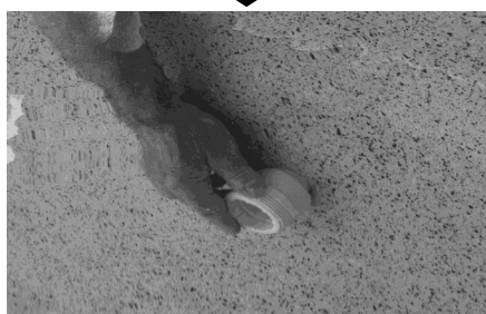
Screw on Insert (3) or (4) firmly
