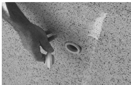
Unscrew ring nut and remove the ball and ring
